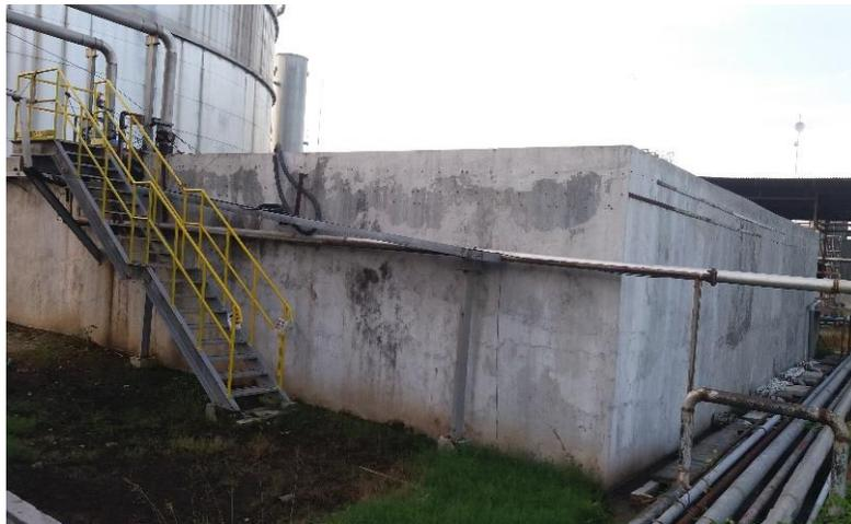
**Gambar 2.2** Kolam presettling
