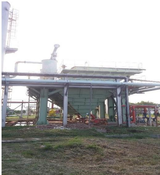
**Gambar 2.5** Lamela degassing pond
